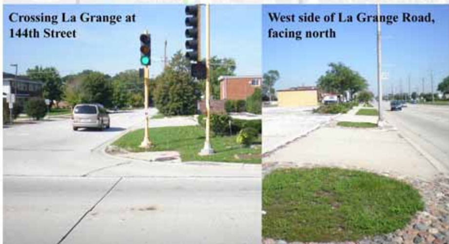
Figure 2 – Existing Conditions North-Center Section: Southwest Highway to 151 st Street
