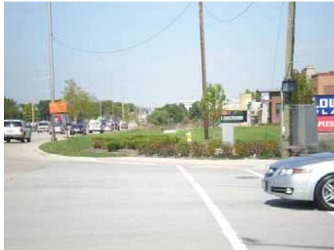
Existing crosswalk terminates into landscaping along La Grange Road at 156 th Street
